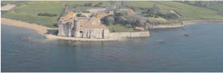
Figure 7 - Some other structures just under the surface of the sea, on the east corner of the castle.
